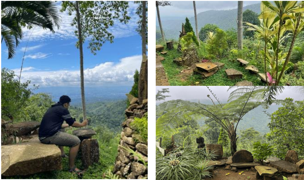
Figure 5. Stone Arrangement and Construction Result
